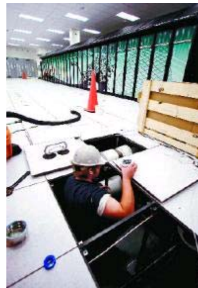
Pipe fitter Bryon Phillips helps
